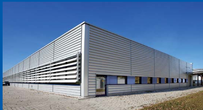
New facility in Markt Indersdorf
